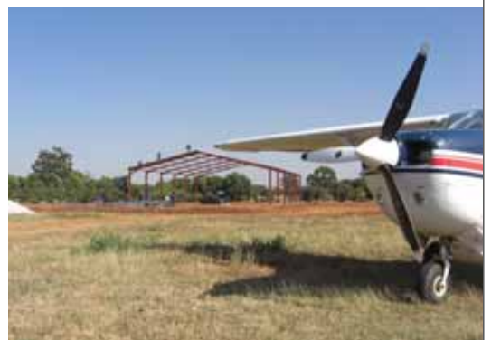
...In Chilongolo a new hangar is being erected...
